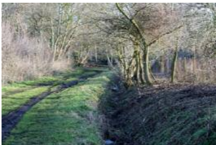
Looking down the short leg of Long Lane from St Michaels Lane, showing removal of trees on the right. 9/2/2010 © HAE Stroude
