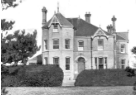
Brookfield House, design resembled that of St Michael's Mount c.1926. Demolished in 1972, to make way for Ladywalk - its entrance followed closely the line of the original drive
