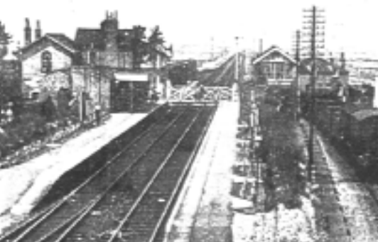
Long Stanton Station, viewed trackside looking towards Swavesey. Middle distance, left to right, main platform, station booking office and house, crossing gates, second platform, signal, signal box and goods siding. Main goods yard was to the left, out of camera. c.1950
